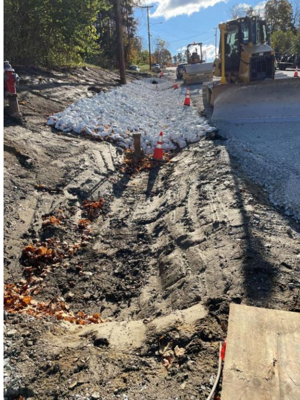
Installation of stone ditching along the southeast side of U.S. 7
