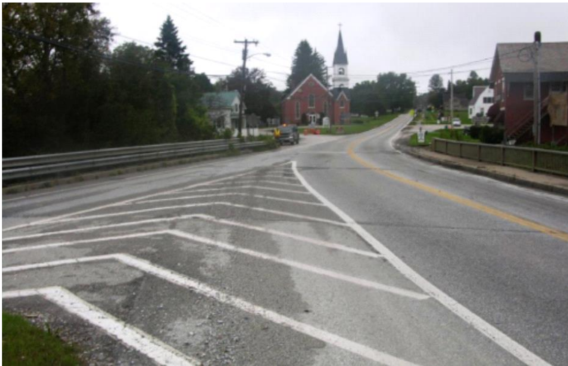
Existing Bridge over the Furnace Brook
