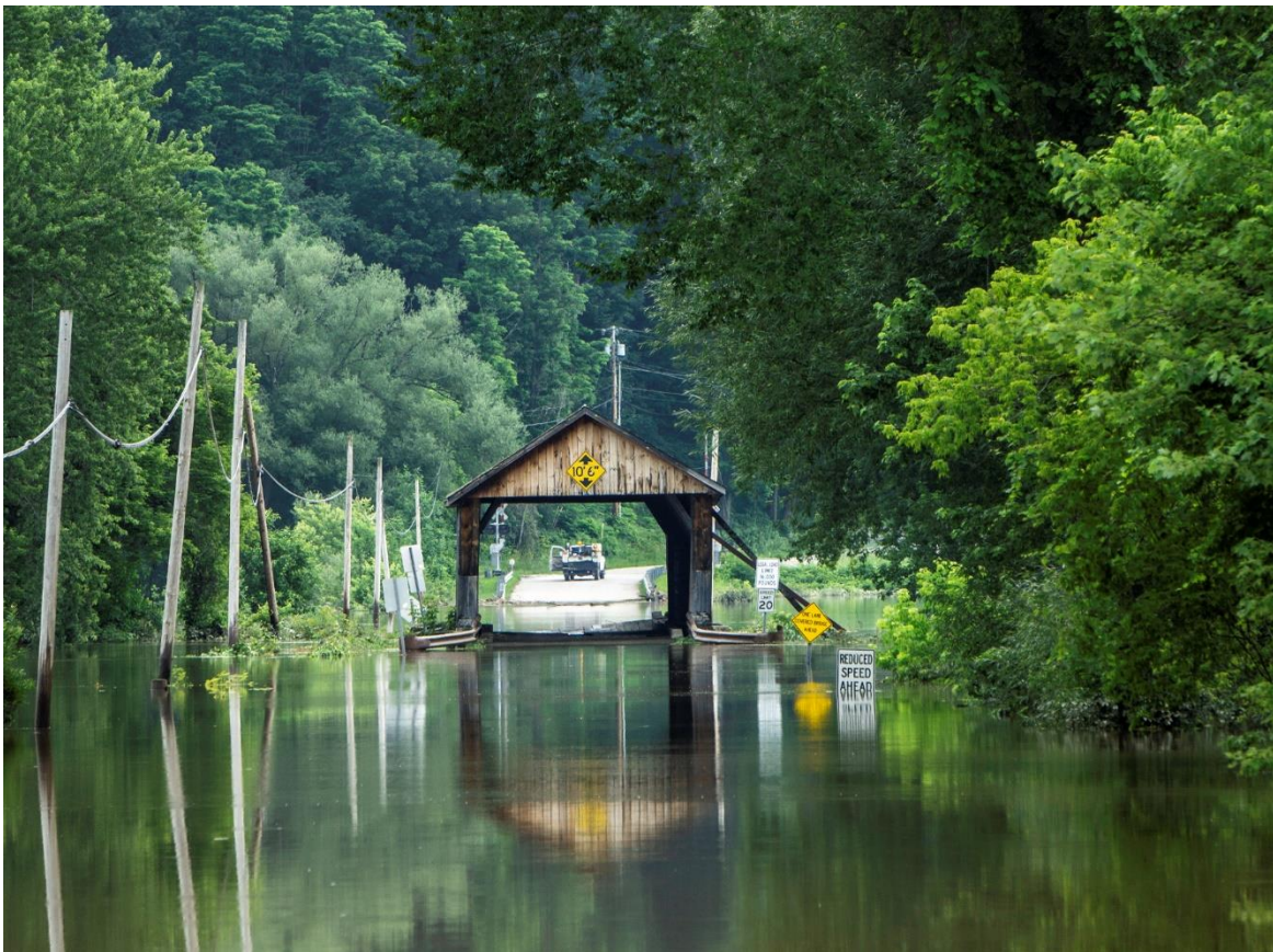
Depot Bridge Flood 2023
